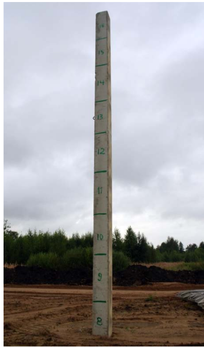
Figure 1 - The pile sticks not reaching target depth.
