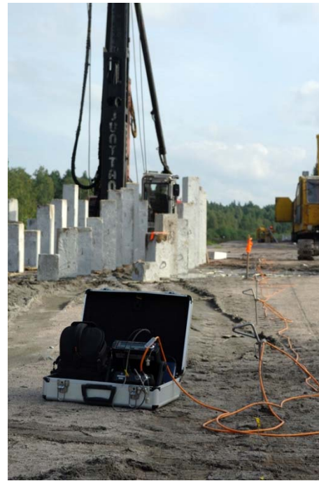
Figure 1 - The pile sticks not reaching target depth.
