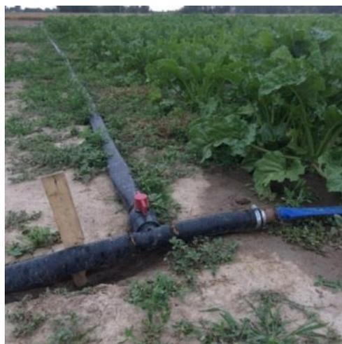
**Figure 6 - Distribution pipes**
