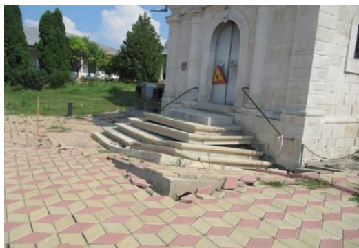
Figure 3 - Highlights the vertical structure disposal/ failure at the porch entrance. The photo is made on 08.08.2014 when was recorded the maximum level of compaction
