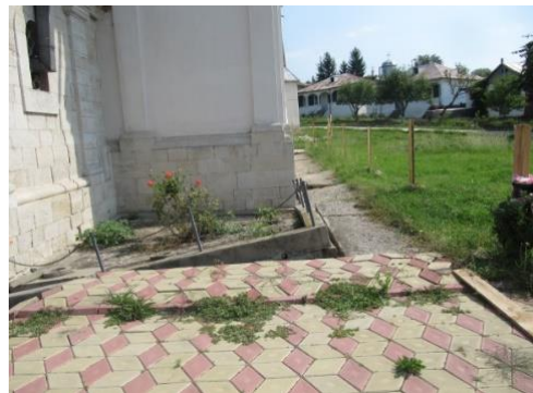
Figure 3 - Highlights the vertical structure disposal/ failure at the porch entrance. The photo is made on 08.08.2014 when was recorded the maximum level of compaction
