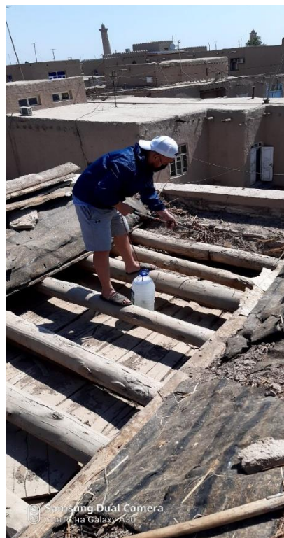
5-picture. Violation of the mosque porch and damage to the roof timber from the termite (processing)
