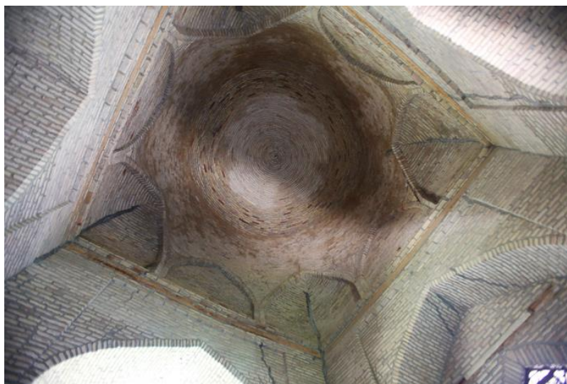
Figure 13 - The dome of the khanaka, on which the grave rests. (Photo by author, 2022)
