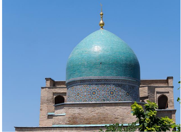
Figure 8 - The turquoise dome stands on a high drum. On both sides are the tops of the stairs, which provide access to small hujras. (Photo by author, 2022)
