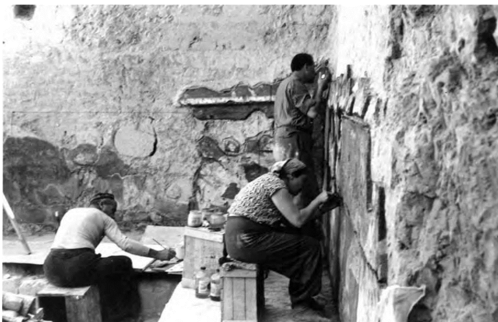
Fig 5. Restorers in process of fixing wall painting layer (source: IICAS,2015)
