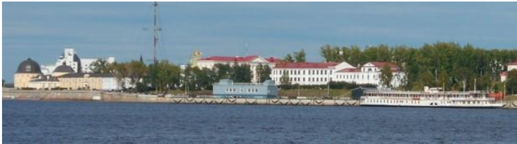
Figure 12. Arkhangelsk. Embankment of the Northern Dvina
