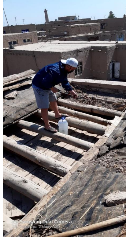
5-picture. Violation of the mosque porch and damage to the roof timber from the termite (processing)
