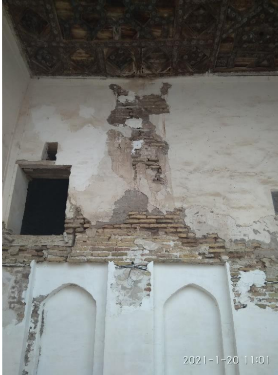
5-picture. Violation of the mosque porch and damage to the roof timber from the termite (processing)
