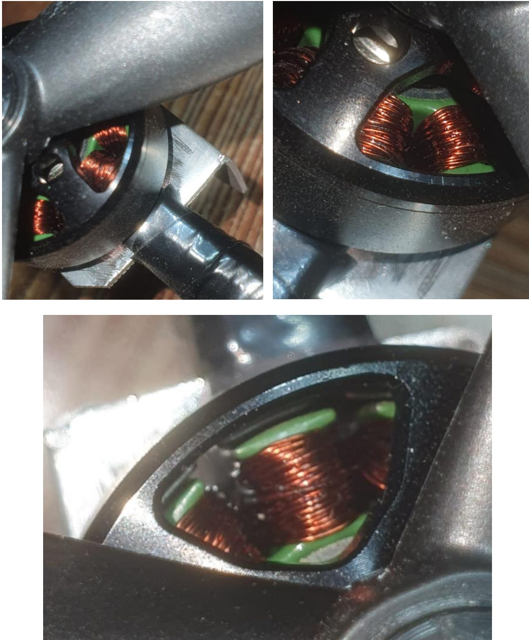
Picture 4. Overheating of the motors.
