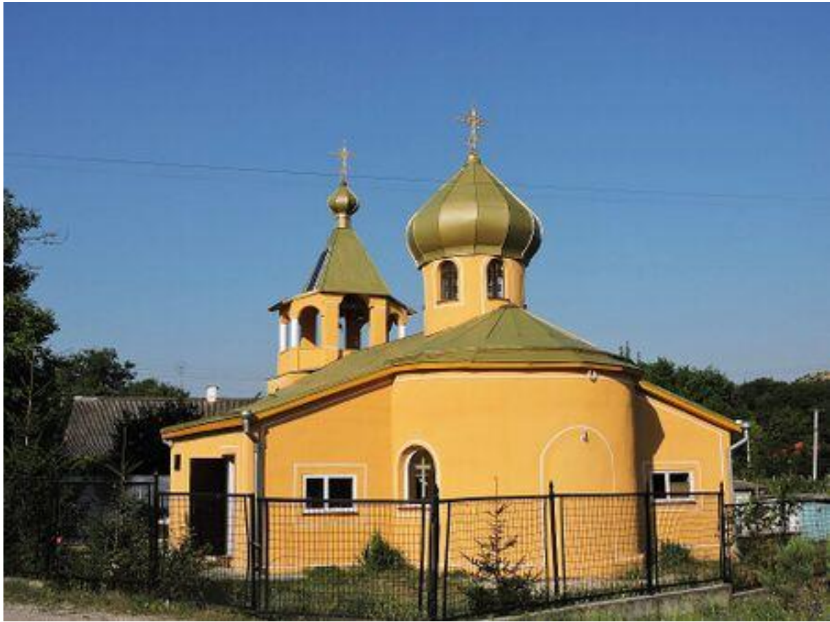
Figure 28. The church was built in 1998 in a store. From 1999 to 2002, the parish completely reconstructed the building into a standard church. The first rector of the church was Hieromonk Abraham. On June 26, 2011, Metropolitan Lazar of Simferopol and Crimea celebrated the Divine Liturgy with the rite of consecration of the altar of the Church of the Nativity of the Prophet Forerunner and Baptist of the Lord John in the village of Khmel'nitskoye. The second rector, for 10 years now, has been priest Vladimir Vorobey. In the Sevastopol deanery, he works with young people, on the Law of God and military-patriotic education. Not far from Khmel'nitskoye, in the village of Oboronnoye, there are healing springs of John the Baptist and the Great Martyr Healer Panteleimon. In the spring of 2012, a carved iconostasis was installed in the church. Currently, the community is raising funds to paint icons for the new iconostasis.
