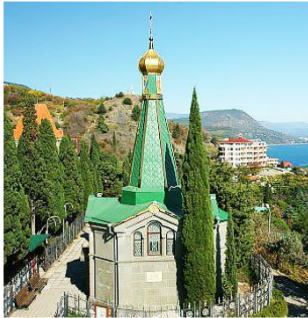
Figure 5. The house church of St. Alexander Nevsky was started to be built simultaneously with the construction of the palace for Princess Anastasia Davydovna Gagarina in 1904-1907. The church, like the palace, was built according to the design of the architect N. P. Krasnov and has an octagonal shape. The corners of the building are cut off, on the northern and southern sides there are three-arched windows, separated by thin columns. A bell tower rises above the church, crowned with a dome with a cross. The mosaic icons were made by academician Shokarev. When a sanatorium was established in the estate in Soviet times, the church was closed.
