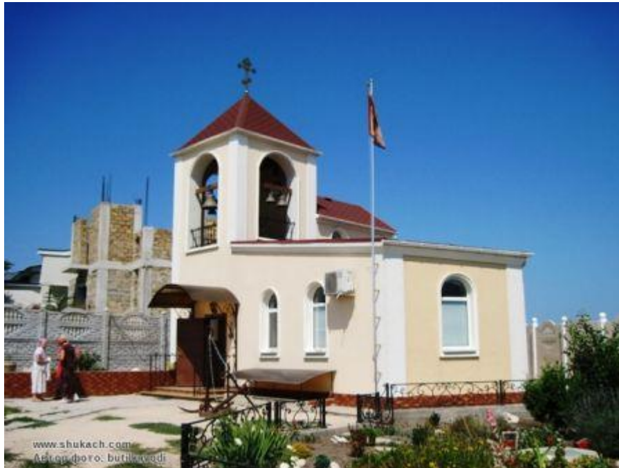
Figure 38. Construction of the Church of the Holy Great Martyr Demetrius of Thessaloniki began on May 13, 2011. At present, a 2-story building with a prayer room and utility rooms, as well as a bell tower, has already been erected using funds from parishioners and benefactors. The parish community plans to build a main, more spacious church and an almshouse. Construction of the almshouse began on November 14, 2014. A sisterhood of mercy was created at the church, the main obedience of which will be serving the residents of the almshouse, organizing and holding charity dinners for the homeless. The first service in the church took place on February 15, 2012, on the feast of the Meeting of the Lord.
