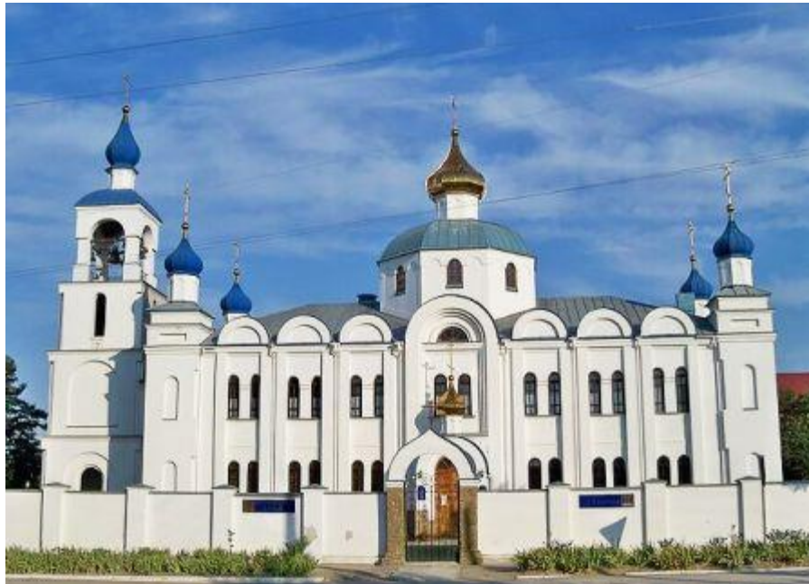
Figure 14. The Church of the Nativity of the Most Holy Theotokos traces its history back to 2000, when the Church was given a civil building at 161 Leo Tolstoy Street, which at various times housed children's institutions: the House of Pioneers, a kindergarten. According to old-timers, in 1938, a representative of the Greek Church consecrated a place for the church where the church is now located. Regular morning prayers and vespers began in September 2000. The religious community "Nativity of the Most Holy Theotokos" was registered on October 24, 2000. The church has two chapels: a church on the second floor in honor of the Nativity of the Most Holy Theotokos, and a church on the first floor in honor of Saint Blessed Xenia of Petersburg. In March 2001, the first Divine Liturgy was celebrated in the lower church. Regular services began. In February 2003, full-scale construction and refurbishment began. The bell tower, drum, main dome and onion were erected. The same year the cross was consecrated and installed. Then the bell tower dome was built. In 2004 the first 5 small bells appeared, on Easter 2005 the blagovest was raised. On the patronal feast day of September 21, 2008 the Divine Liturgy was served in the upper church for the first time.
