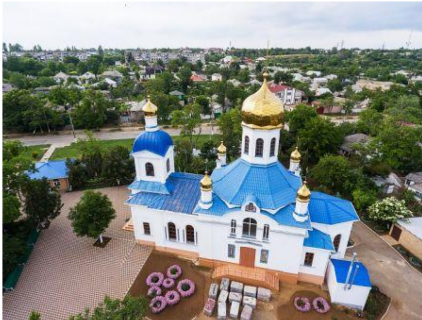
Figure 17. Before the construction of their own church, Orthodox residents of the village of Stary Karantin (now the Arshintsevo district) had to travel along dirt roads to the center of Kerch to attend services, where the nearest Alexander Nevsky Church was located. In the fall of 1903, State Councilor Alexander Vasilyevich Novikov donated a plot of his land to the city, and he donated part of it, in the center of the village, on a hill, for the construction of the church. On June 18, 1904, the project by the provincial architect A. Karapetyan was approved, and on August 1, 1905, construction of the church began with funds from the residents of this village. On February 5, 1907, a relatively small church with a height of 18.1 m, designed for 350-450 people, was consecrated in honor of the Ascension of the Lord. It had three entrances, 15 windows, a stone three-tiered bell tower 19.2 m high. The central drum, bell tower and four cupolas were crowned with helmet-shaped domes. Inside there was a wooden iconostasis covered with brown varnish, and the church yard was surrounded by a stone fence.
