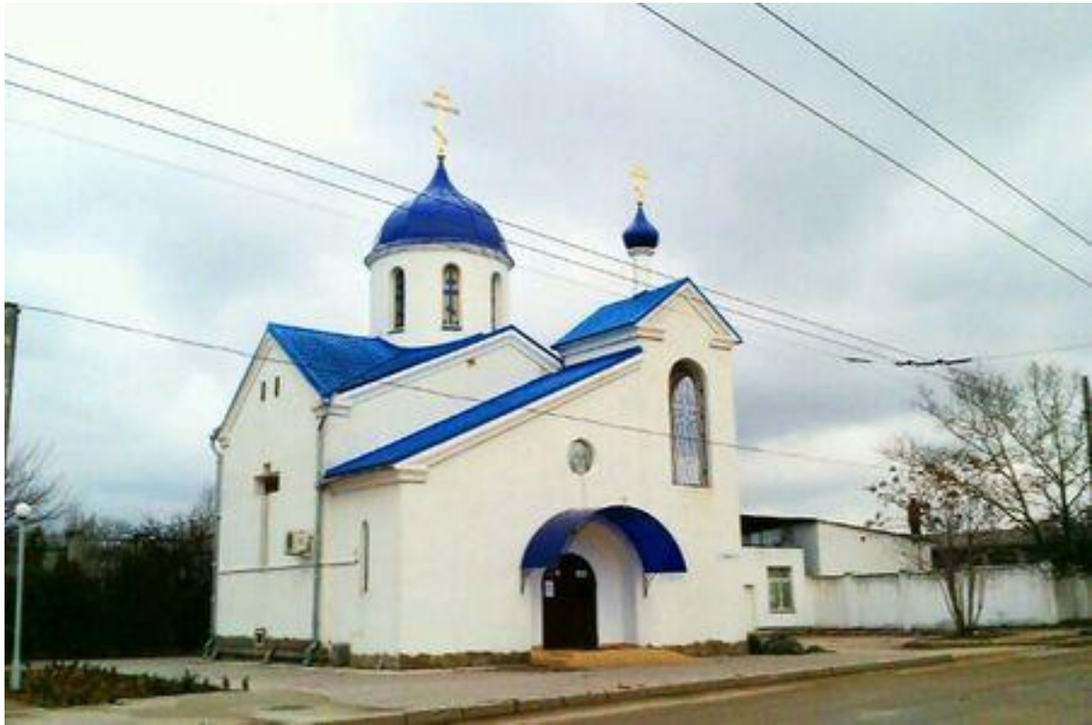
Figure 32. The temple was built with funds from the Sevastopol Dairy Plant, the idea of construction belongs to its owner Sarkisov A.A. The temple is located directly next to the entrance of the plant next to the trolleybus stop. Small in appearance, quite roomy inside. Since January 1, 2012, after repairs, services have been resumed in the temple in the name of the icon of the Mother of God "Joy of All Who Sorrow".
