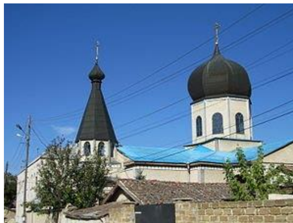
Figure 2. The St. Nicholas Church in Belogorsk traces its history back to 1793, when a Greek cathedral in the name of St. Nicholas was built in Karasubazar (as Belogorsk was called until 1944). The construction of the church was blessed by His Grace Job (Potemkin), Bishop of Feodosia and Mariupol. Infantry General Count M. V. Kakhovsky and parishioners provided considerable assistance. Over the course of its history, the church has been rebuilt several times: an extension was gradually added, the wooden bell tower was replaced by a stone one, and the building acquired features of the Byzantine style. The first cathedral archpriest was John Vasilkioti, who served here for about 50 years, until the end of his life. According to Bishop Hermogenes, he was highly respected not only by the Greeks, but also by the Tatars.
