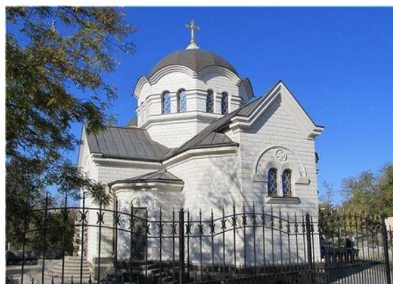
Figure 24. The Church of the Ascension of the Lord is a stone church built in 1903-1905 in memory of the successful retreat of the Russian army to the Northern side of Sevastopol during the abandonment of the
