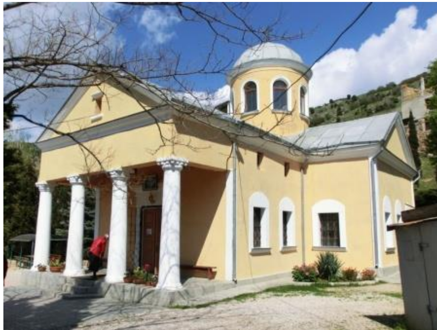
Figure 25. The Church of the Holy Twelve Apostles in Balaklava, along with other Orthodox churches in Crimea, is a unique architectural monument of the 18th century. It was erected in the name of St. Nicholas the Wonderworker in 1794. The construction material was rubble limestone mined in the stone quarries of Crimea, and the building itself was erected on the foundation of an ancient church built here in 1375. In 1861, during reconstruction work on the church, a stone was discovered above its entrance, hidden under a layer of plaster, with an inscription reading: "1357, on September day, this construction was begun during the reign of the humble man Simone de Orto, consul and castellan." Genoese craftsmen left such stone boards in the buildings they built. According to researchers, the stone with the inscription was used a second time during the construction of the Church of the Holy Twelve Apostles.
